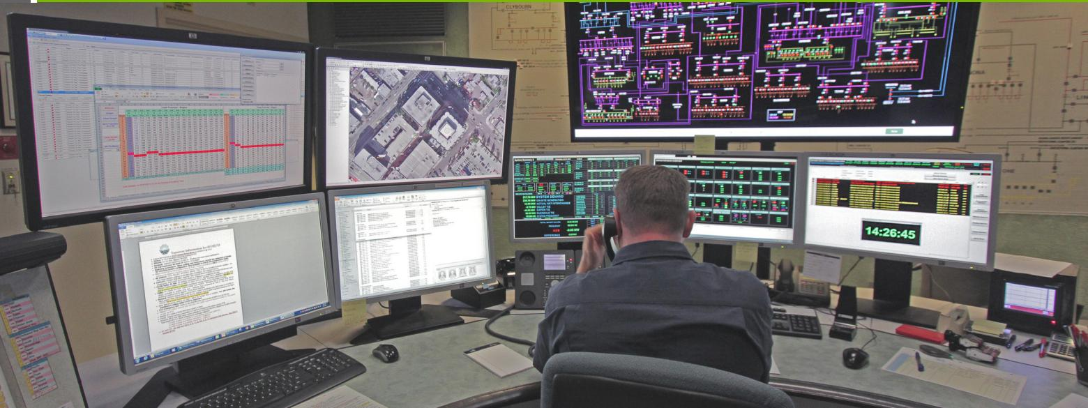
Landis+Gyr's Transmission and Distribution SCADA software (TDS) simplifies the management of both large and small utility control centers. The solution is a distributed client/server SCADA system that supports multiple front-end processors, servers, and operator workstations. It includes voice synthesis, areas of responsibility, automatic alarm inhibit, customizable alarm sounds, and other advanced functions.
